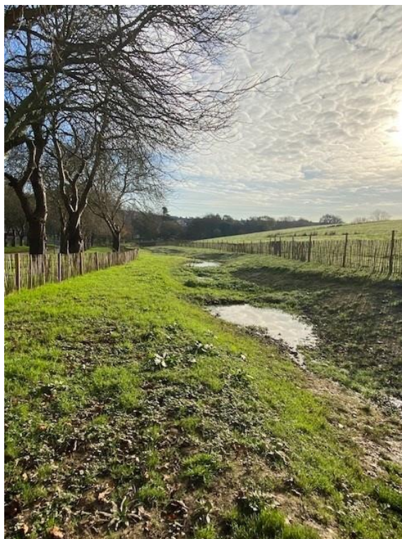
Picture 4 - Swale – showing new fencing position tight to the swale.
